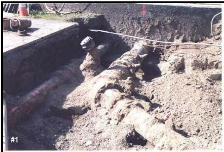
Photograph 1: Before below-ground retrofit
