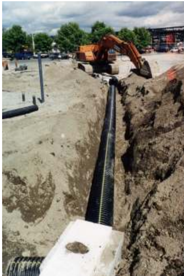
Photograph 5: New fuel lines installed. Source: Port of Edmonds
