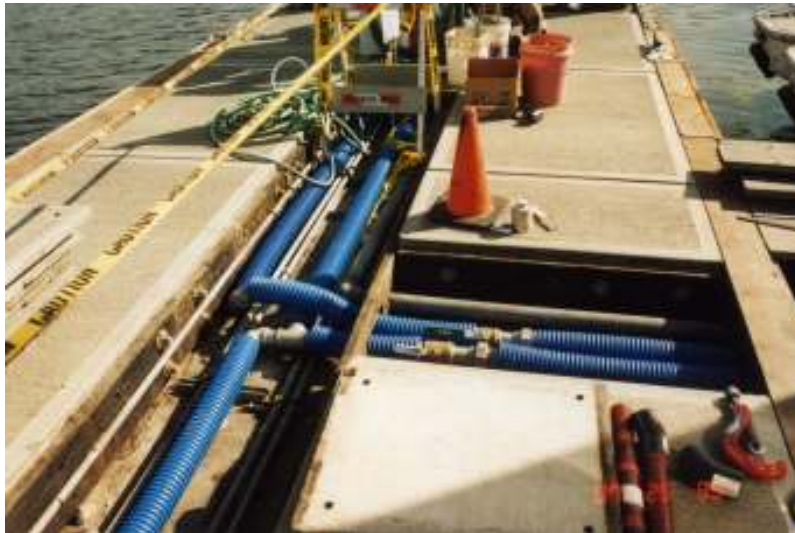
Photograph 3: New dock and embedded fuel lines.
