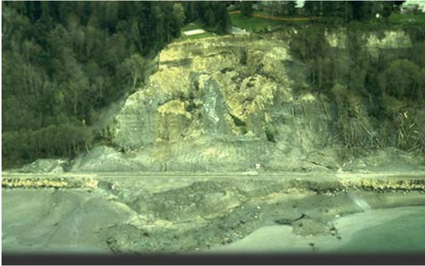
Figure 1: Woodway Landslide, January 15, 1997.
